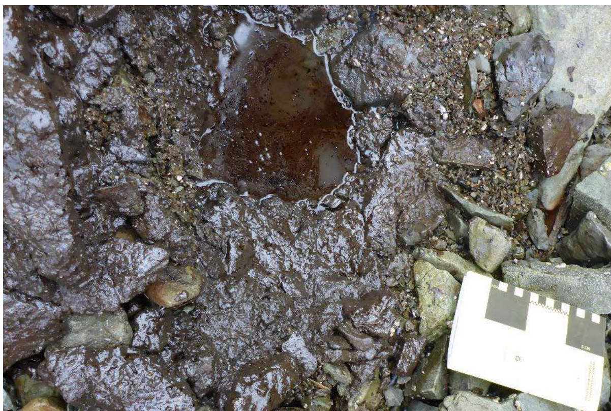
Figure B.7 EL-056C pit at WP 8 with brown oil
